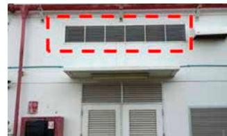
Improvement of compressor room air intake (Thailand)
