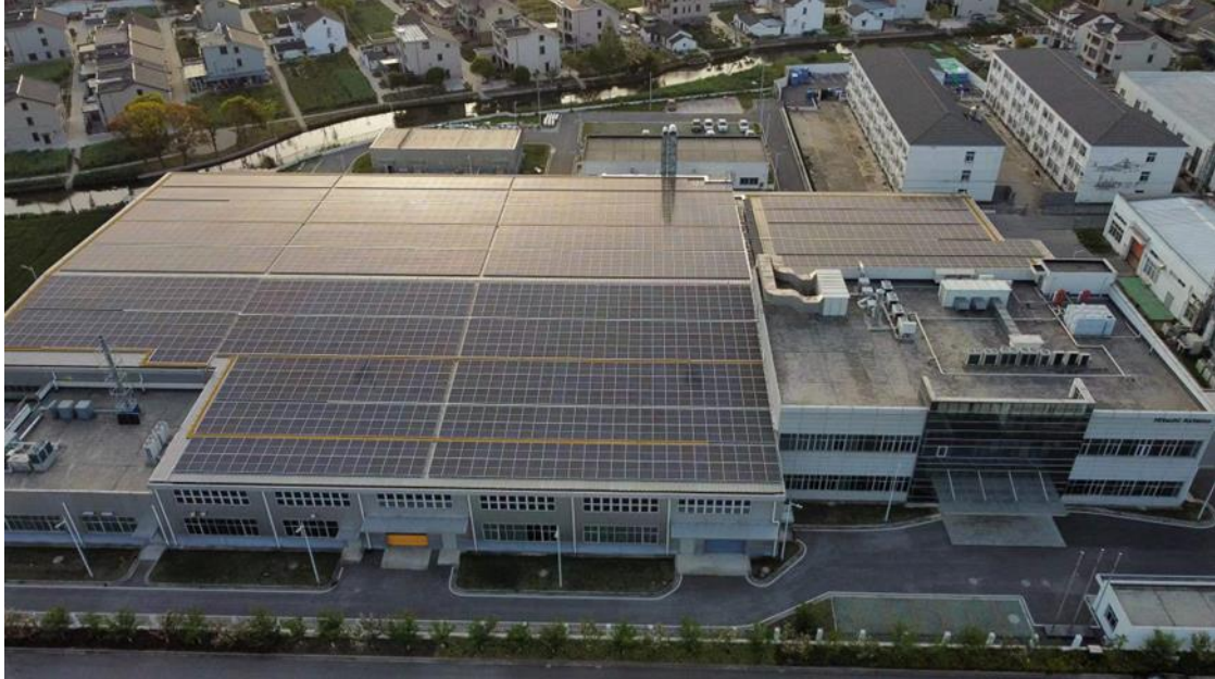
Solar panels installed on Hitachi Astemo train system (Changshu)
