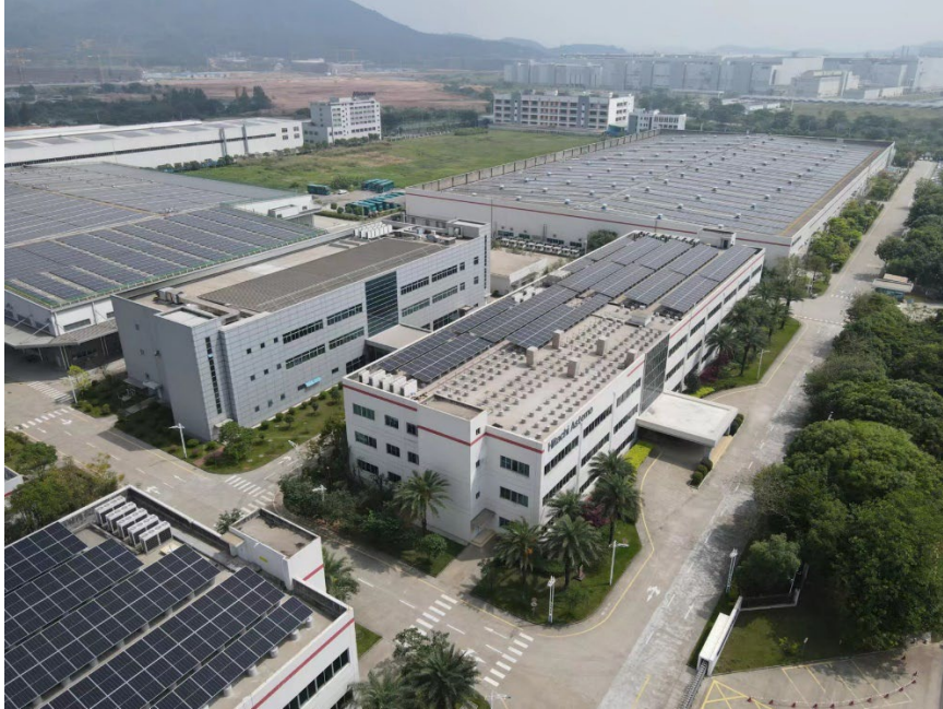
Solar panels installed at Hitachi Astemo Automotive Systems (Guangzhou)
