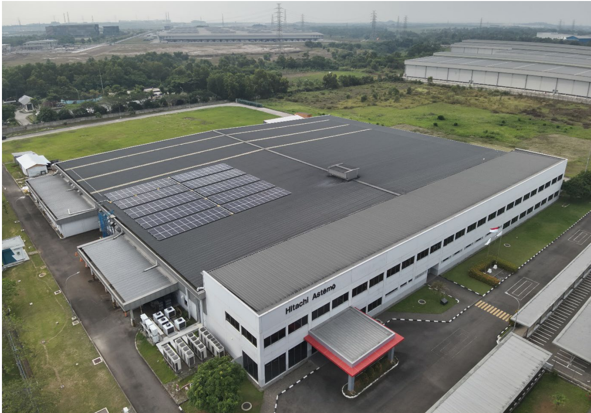
Solar panels on the roof of Bekasi Plant #2
