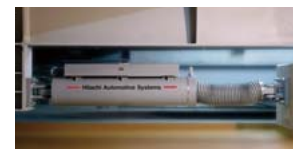
Seismic Isolation Oil Dampers
